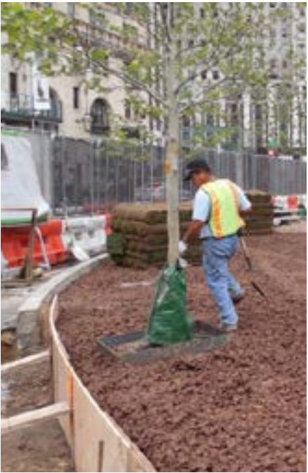
Structural Soil Install
